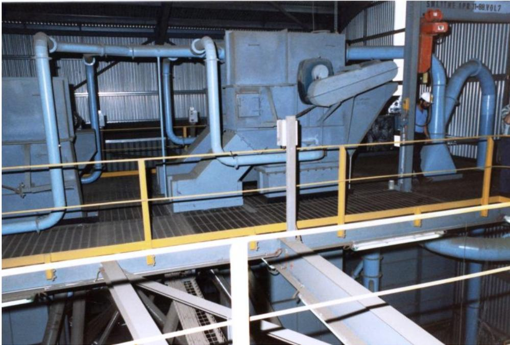
Figure B.12.: Insulation around gravity discharge pipes – assists in minimising thermal convections
