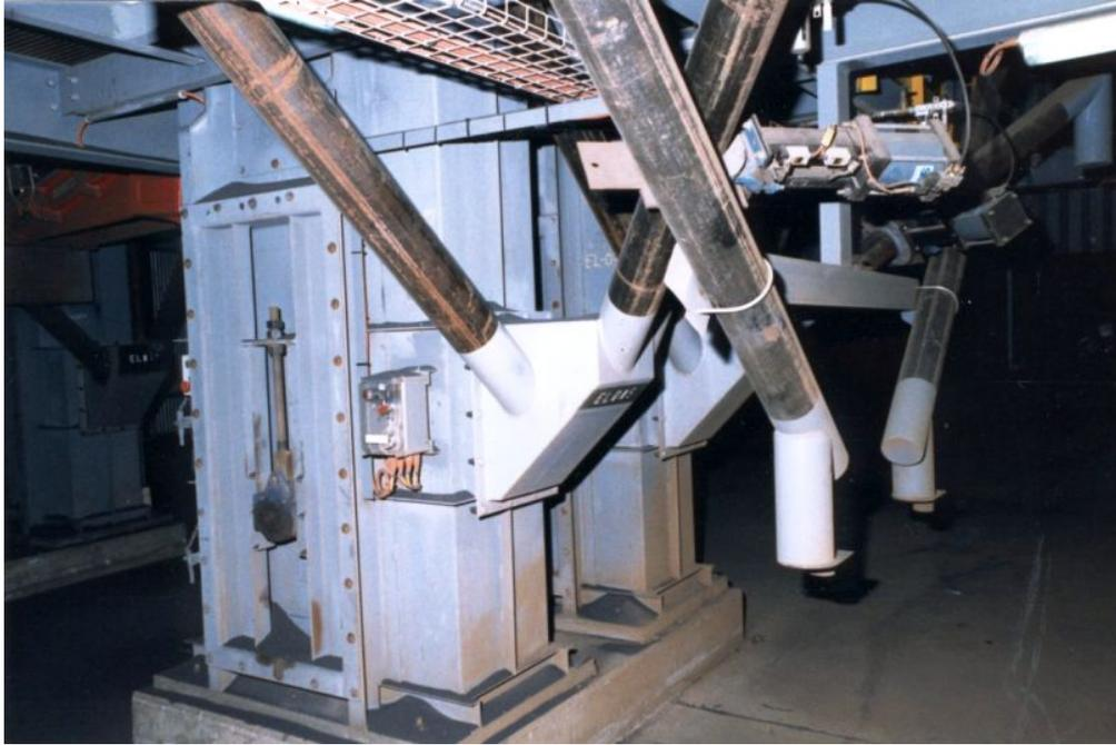
Figure B.10.: Open mesh cable trays – minimises dust accumulation
